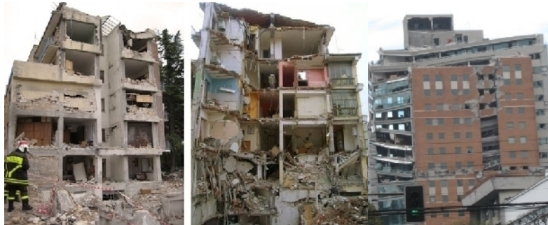
Figure 1. Reinforced concrete frames damaged in L'Aquila earthquake 6th of April 2009 and Chile earthquake 27th of February 2010
