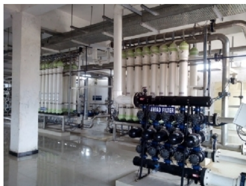
Figure 2. Amiad Filter & Ultra-filter (UF)
