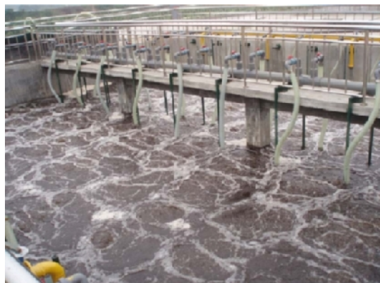
Figure 3. Submerged Membrane Bioreactor
