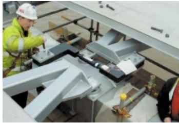
Figure 1. Installation of viscous dampers beneath the deck of the London Millennium Bridge
