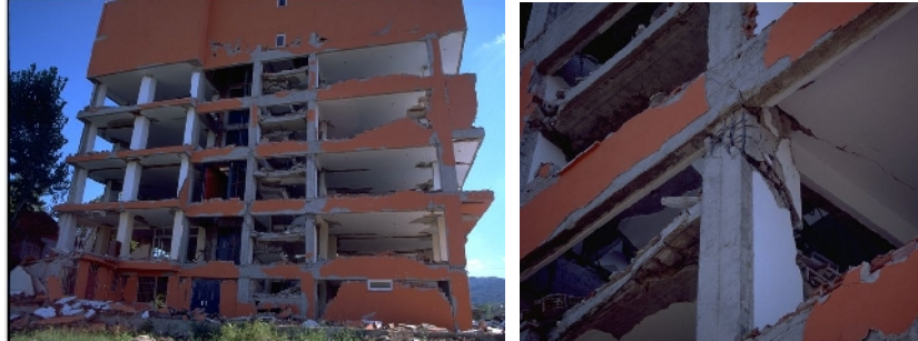
Figure 1. Damaged RC frame with hollow clay tile infill masonry, Izmit 1999 (Elwood et al. , 2000)
